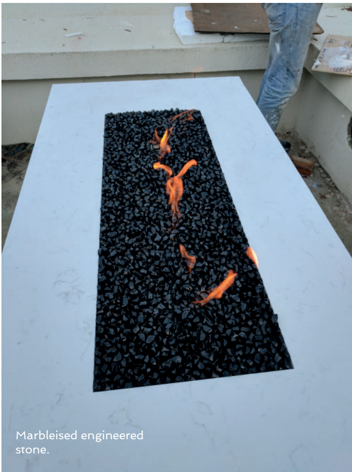
Engineered stone on a masonry base.
